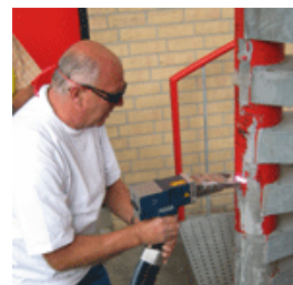
Laser Paint Stripping
