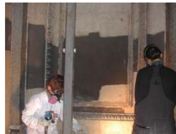
Sandstone Wall During Cleaning
