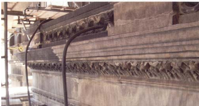
Foreground detail after start of Laser Cleaning
