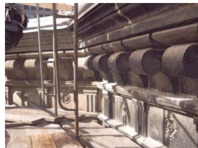
Historic Building Laser Cleaned in Background
